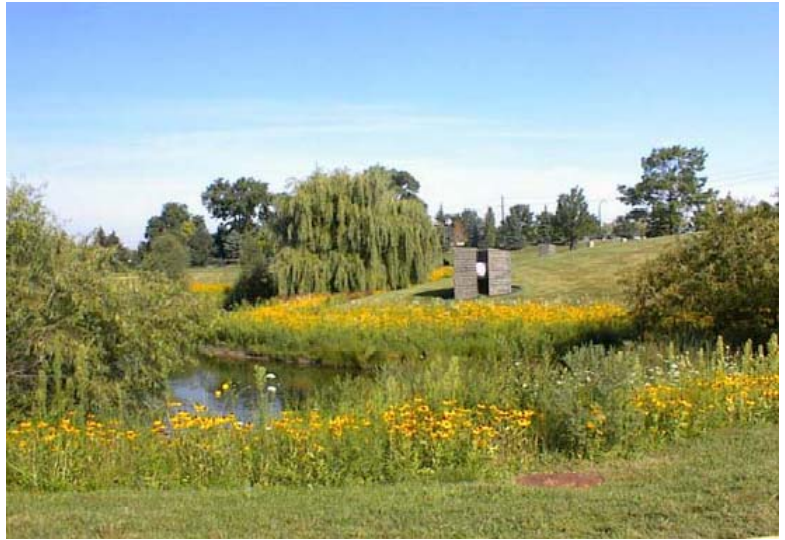
This stormwater pond is located at the Pfizer Global Research and Development facility in Ann Arbor. This is a beautiful example of a pond buffer created with native plants.
