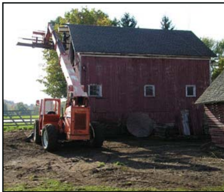
Repairs being completed on one of the historic barns
