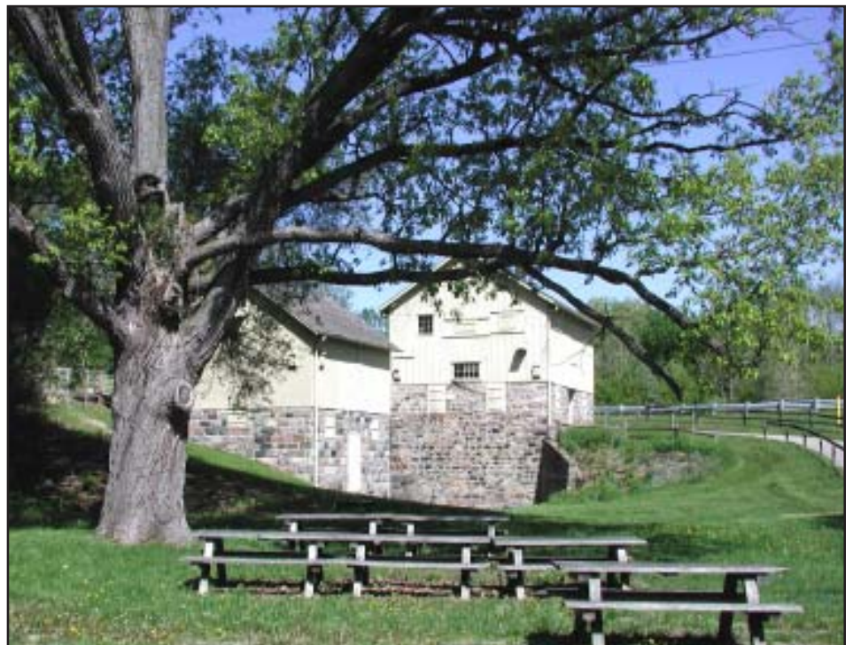
Today the Parker Mill buildings appear relatively unchanged from the late 1800s. In fact, new structural beams, siding and roofs, and conversion to an electric-powered turbine were among the extensive renovations commissioned by WCPARC in 1983. Historical authenticity was ensured by Amish craftsmen.
