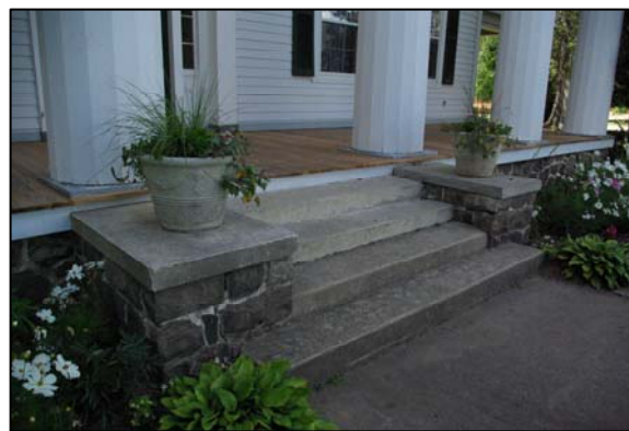
Gordon Hall's New Front Porch Decking
