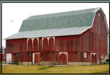
Gambrel asphalt shingle roof, 14470 Allan Road, Bridgewater Township
