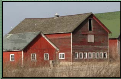
Cody Barn with wood shingle gable roof 670 Textile Road, Pittsfield Township
