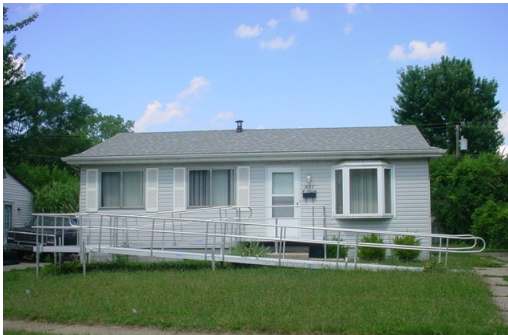
Wheelchair ramp installation in Ypsilanti
