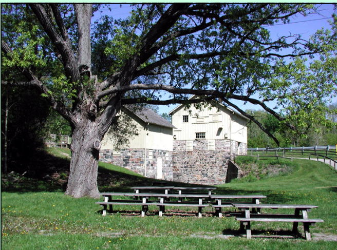
Historic structure at Parker Mill County Park in Ann Arbor Township; Connected to Gallup Park by a recreational path.
